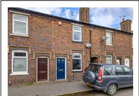
High Street, Wollaston, Stourbridge
