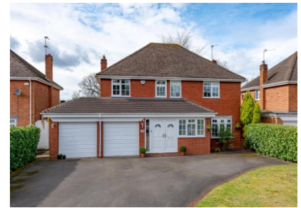
18 Corfton Drive, Tettenhall
