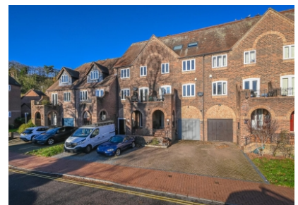
22 Southwell Riverside, Bridgnorth
