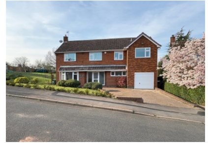
Tanglewood, 12 The Wold, Claverley, Shropshire
