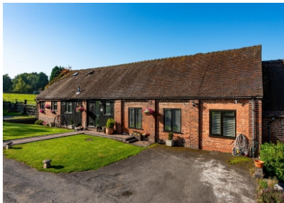
Barn End, Codsall Road, Palmers Cross, Wolverhampton
