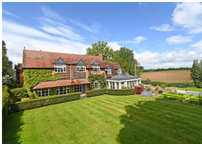
The Gate House, Sandford, Claverley, Wolverhampton
