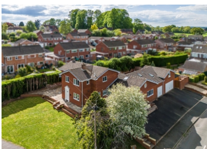
Corner House & Annexe, Daddlebrook Road, Alveley, Bridgnorth
