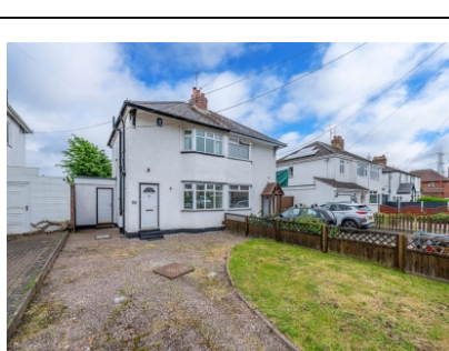
Brickbridge Lane, Wombourne, Wolverhampton
