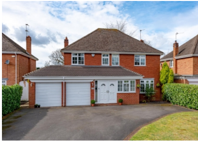
18 Corfton Drive, Tettenhall
