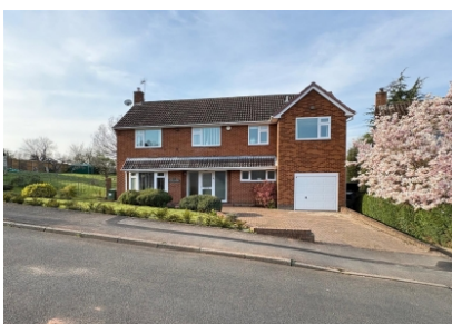
Tanglewood, 12 The Wold, Claverley, Shropshire
