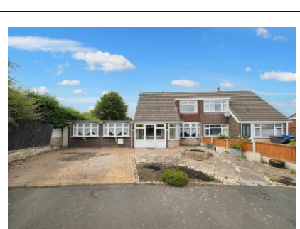
Greenfields Road, Wombourne, Wolverhampton
