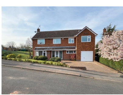
Tanglewood, 12 The Wold, Claverley, Shropshire
