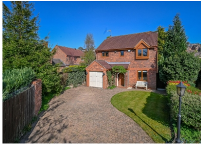
4 Washbrook Road, Bridgnorth,
