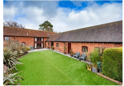
Clee View Barn, Westbeech Road, Patttingham, Wolverhampton
