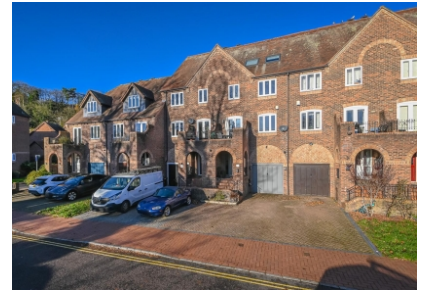
22 Southwell Riverside, Bridgnorth
