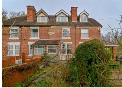
3 The Elms, Station Road, Highley, Bridgnorth
