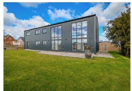
Coppice View Barn, Glazeley, Bridgnorth
