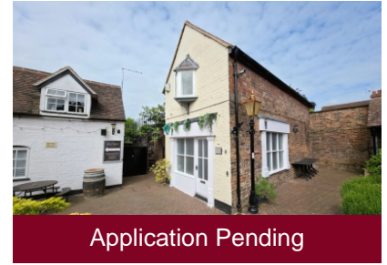
Flat 10 Central Court, High Street, Bridgnorth
