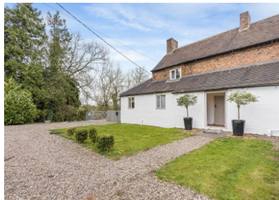
Blythbury Farmhouse Cottage, Shifnal
