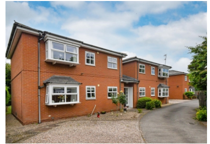
Maypole Court, Gravel Hill, Wombourne, Wolverhampton
