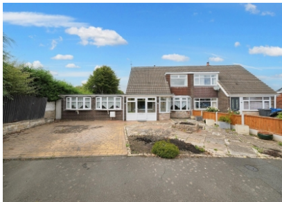
Greenfields Road, Wombourne, Wolverhampton
