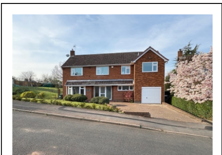
Tanglewood, 12 The Wold, Claverley, Shropshire
