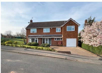
Tanglewood, 12 The Wold, Claverley, Shropshire
