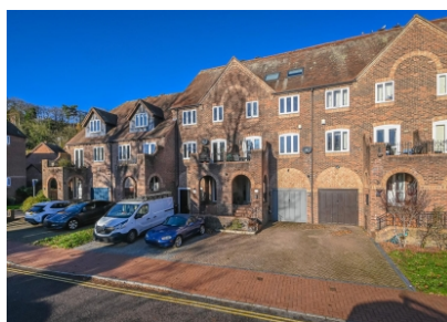
22 Southwell Riverside, Bridgnorth
