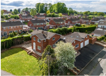
Corner House & Annexe, Daddlebrook Road, Alveley, Bridgnorth
