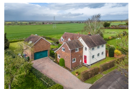
Underhill, 14 Charlton, Telford
