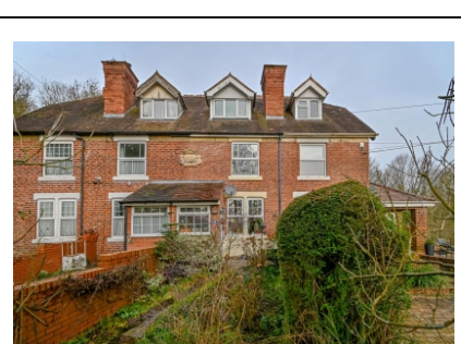
3 The Elms, Station Road, Highley, Bridgnorth
