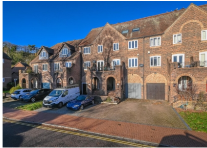
22 Southwell Riverside, Bridgnorth
