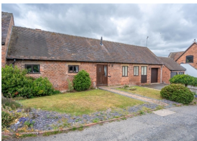
Rosemary Cottage, Codsall Road, Tettenhall, WV6 9QG
