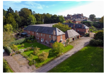
The Bothy (and Barns for conversion), Patshull Park, Patshull Hall, Burnhill Green, Wolverhampton
