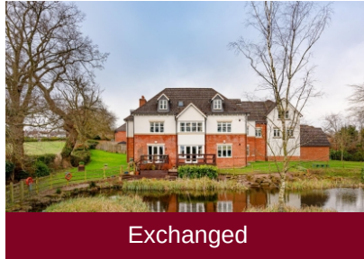
4 Albrighton House, The Water Gardens, Wolverhampton
