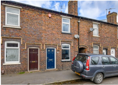
High Street, Wollaston, Stourbridge
