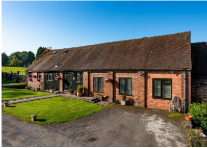
Barn End, Codsall Road, Palmers Cross, Wolverhampton
