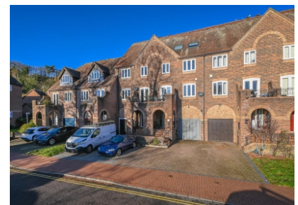
22 Southwell Riverside, Bridgnorth
