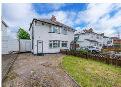
Brickbridge Lane, Wombourne, Wolverhampton
