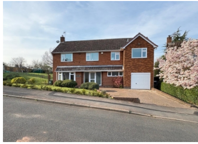
Tanglewood, 12 The Wold, Claverley, Shropshire
