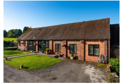
Barn End, Codsall Road, Palmers Cross, Wolverhampton
