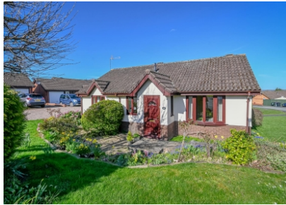
14 Fairfield, Bridgnorth, Shropshire
