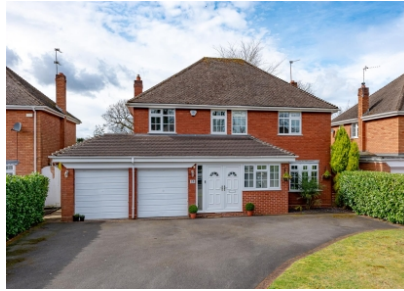
18 Corfton Drive, Tettenhall
