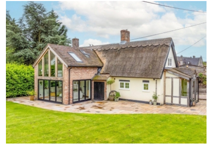
Worthington Cottage, 24 Village Road, Norton, Shifnal
