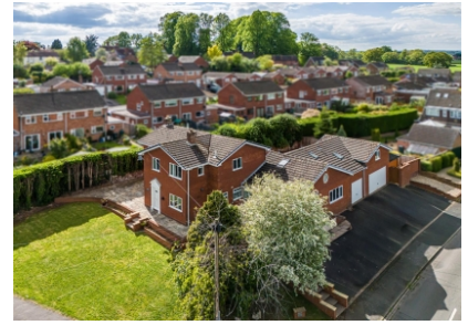
Corner House & Annexe, Daddlebrook Road, Alveley, Bridgnorth
