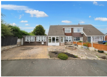
Greenfields Road, Wombourne, Wolverhampton
