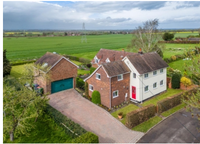
Underhill, 14 Charlton, Telford
