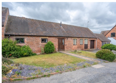
Rosemary Cottage, Codsall Road, Tettenhall, WV6 9QG
