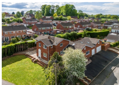
Corner House & Annexe, Daddlebrook Road, Alveley, Bridgnorth
