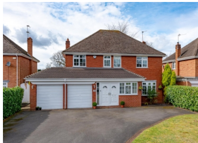
18 Corfton Drive, Tettenhall
