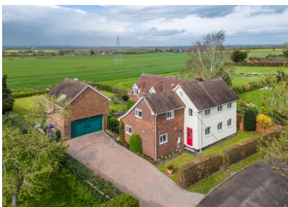
Underhill, 14 Charlton, Telford
