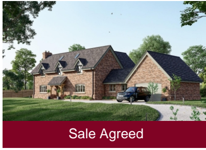
Building Plot, Middle House, Corfton, Craven Arms
