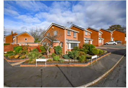
Carnforth Close, Kingswinford
