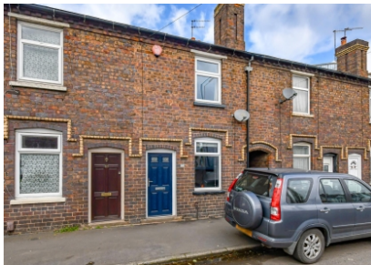
High Street, Wollaston, Stourbridge
