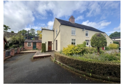
37a Mount Road, Tettenhall Wood
