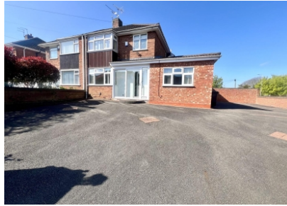
37 Ennerdale Road, Tettenhall, Wolverhampton
