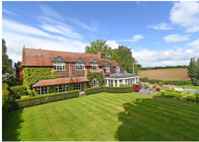
The Gate House, Sandford, Claverley, Wolverhampton
