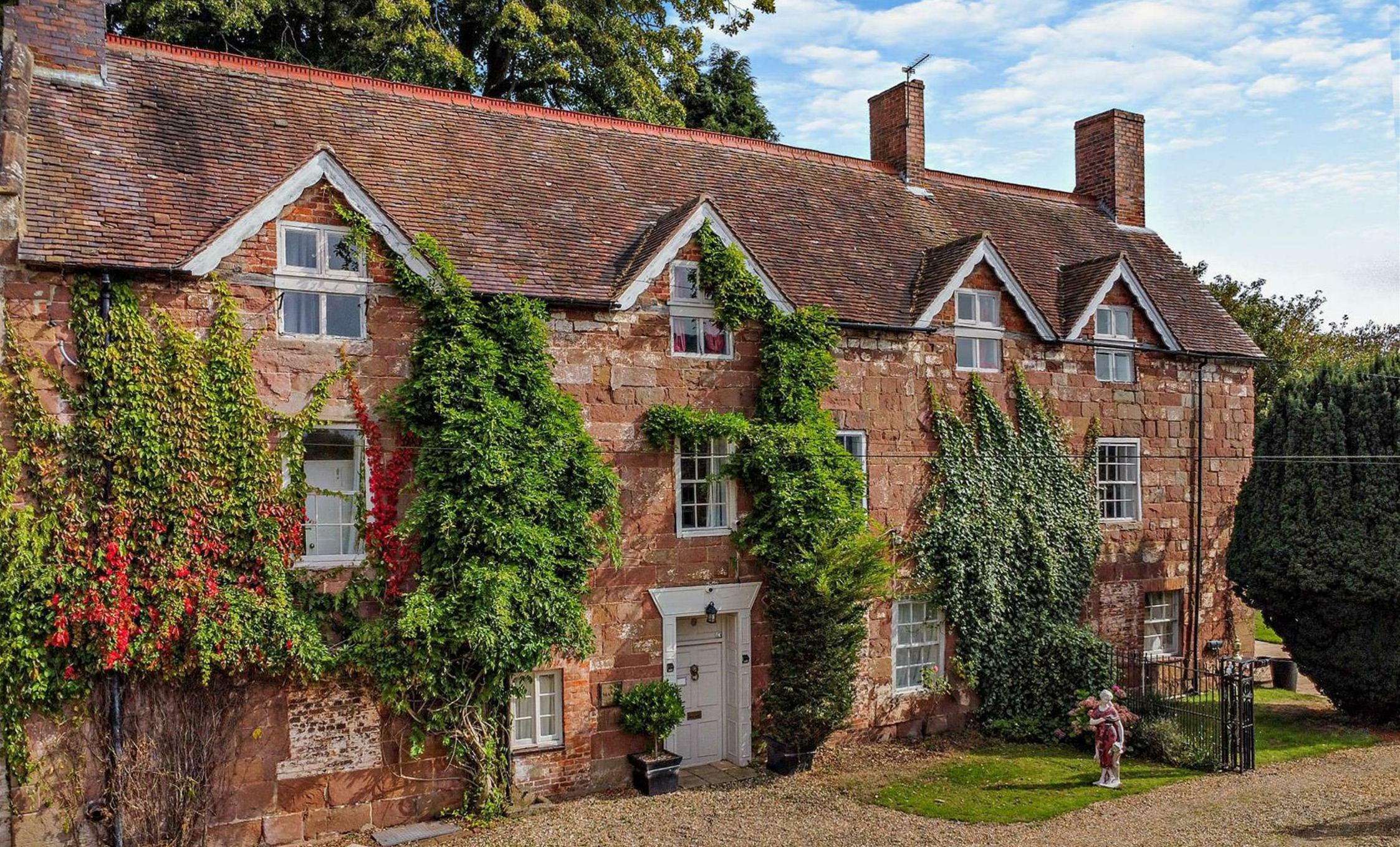
Manor House, Manor, Shifnal, Shropshire, TF11 9PB
