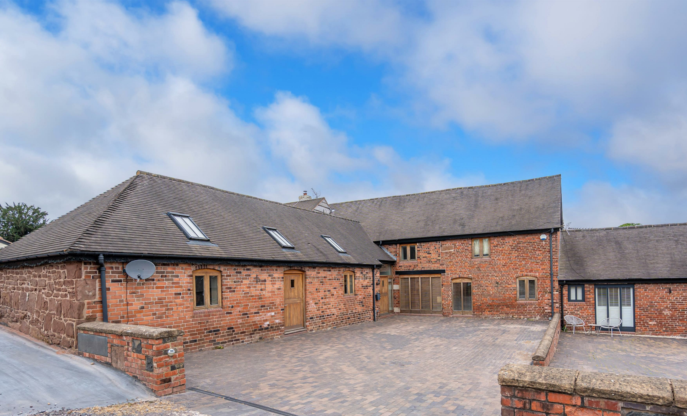
Barn 1 Knowle Bank Farm, Knowles Bank, Shifnal, TF11 9PG
