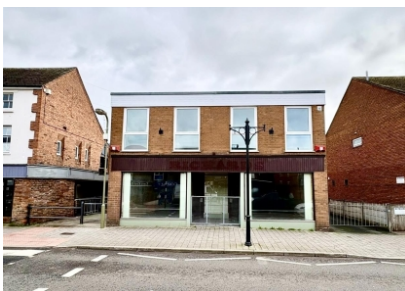
8a Bradford Street, Shifnal
