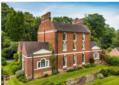
The Dower House and Coach House, Hollybush Lane, Codsall, South Staffordshire, WV8 2AT
