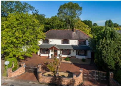
Highcroft, Holyhead Road, Albrighton, Wolverhampton, WV7 3AN
