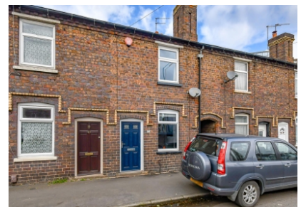
High Street, Wollaston, Stourbridge
