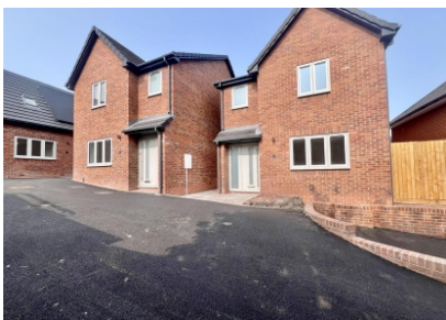
1 Bull Lane, Link Road, Wombourne
