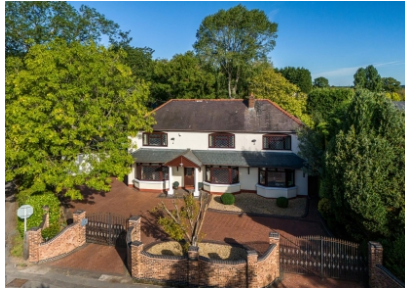
Highcroft, Holyhead Road, Albrighton, Wolverhampton, WV7 3AN
