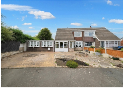
Greenfields Road, Wombourne, Wolverhampton
