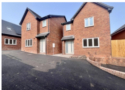
2 Bull Lane, Link Road, Wombourne
