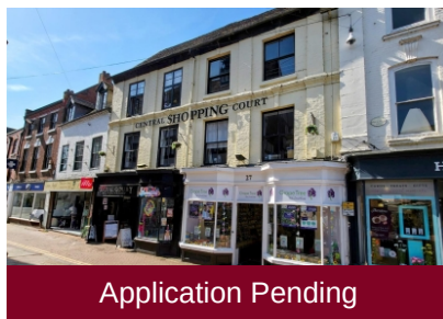
Flat 2, Central Court, High Street, Bridgnorth
