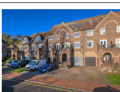
22 Southwell Riverside, Bridgnorth
