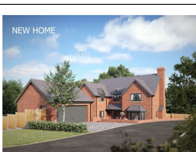
5 The Stamp Works, Ludlow Road, Bridgnorth
