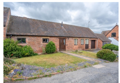
Rosemary Cottage, Codsall Road, Tettenhall, WV6 9QG
