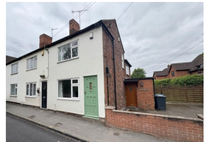
3 Giggety Cottages, Wombourne
