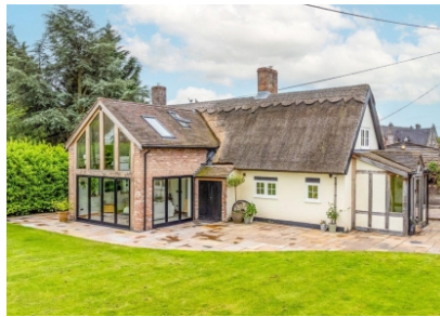
Worthington Cottage, 24 Village Road, Norton, Shifnal
