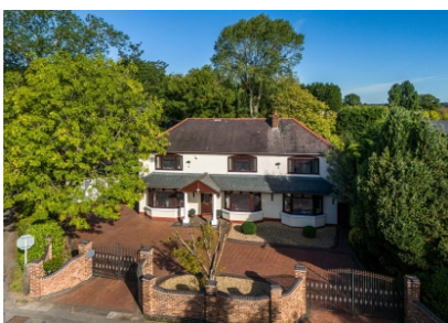
Highcroft, Holyhead Road, Albrighton, Wolverhampton, WV7 3AN
