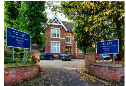
Apartment 11 Beacon House, Tettenhall Road, Newbridge
