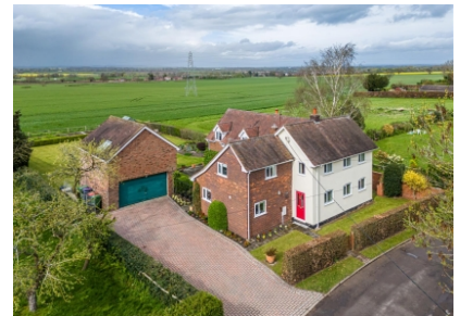
Underhill, 14 Charlton, Telford
