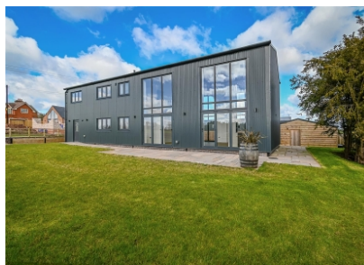
Coppice View Barn, Glazeley, Bridgnorth
