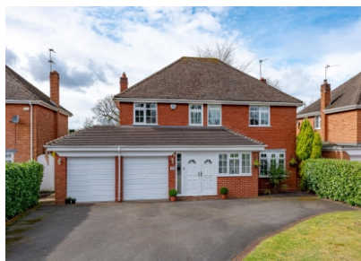
18 Corfton Drive, Tettenhall
