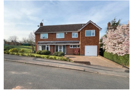
Tanglewood, 12 The Wold, Claverley, Shropshire
