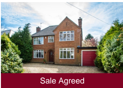
115 Wrottesley Road West, Tettenhall, Wolverhampton, WV6 8UP
