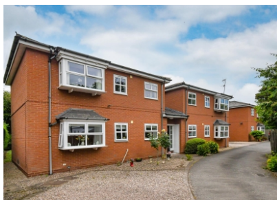
Maypole Court, Gravel Hill, Wombourne, Wolverhampton
