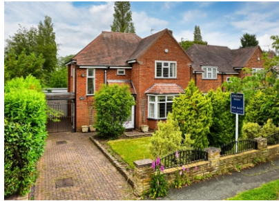
40 Cranford Road, Finchfield, Wolverhampton, WV3 8EP
