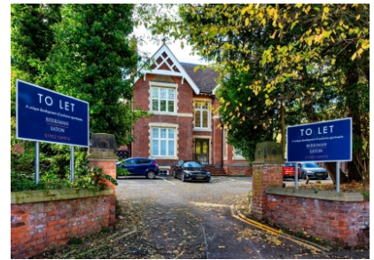
Apartment 2 Beacon House, 267 Tettenhall Road
