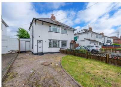
Brickbridge Lane, Wombourne, Wolverhampton
